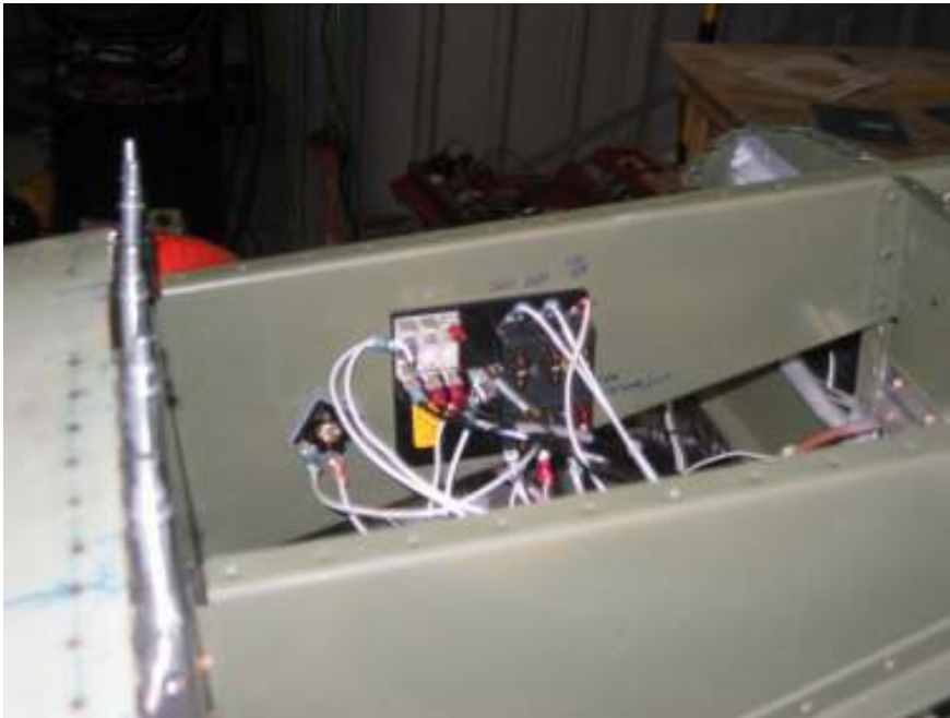
Move E-bus back to panel support and rewire
