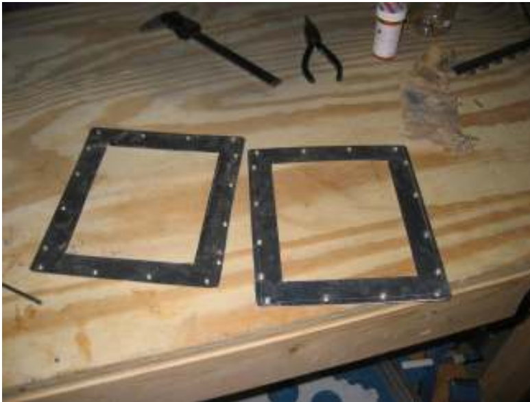
Cut front deck access panel to replace is center with fiber glass Total time: 6 hours (1035 hrs)
