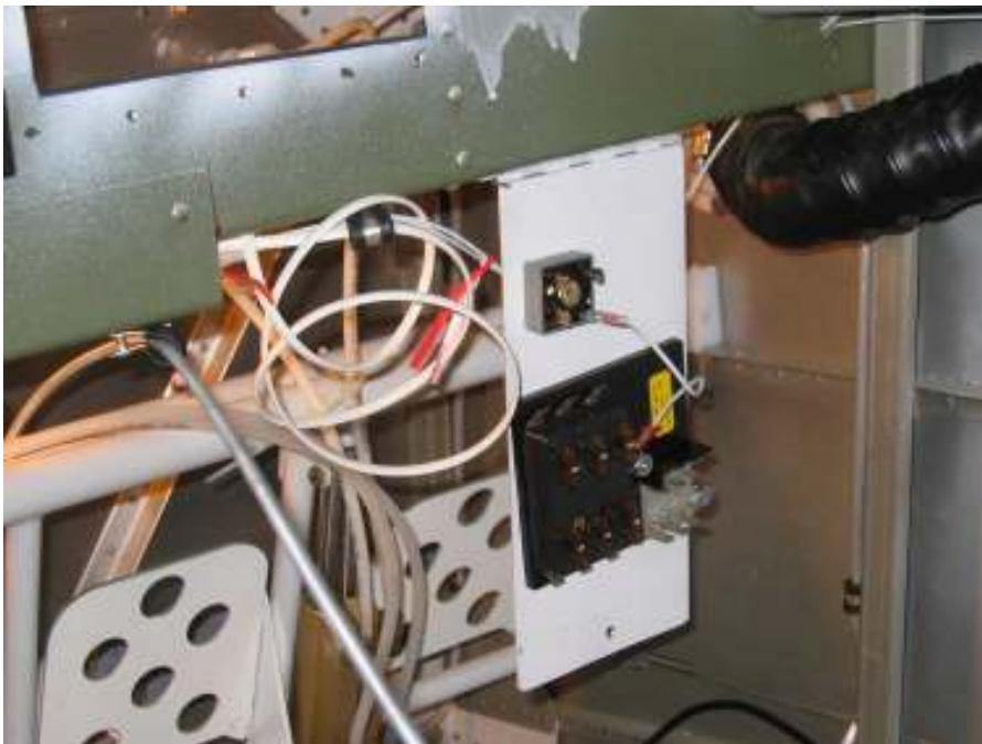
Mount e-bus tray to the subpanel and relocate e-bus and diode to the tray, install nutplate on panel for the tray Determine parking brake control location and mounting bracket
