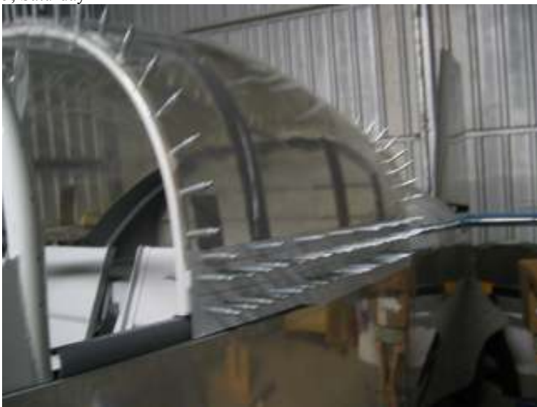
Drill canopy skirt to the frame
