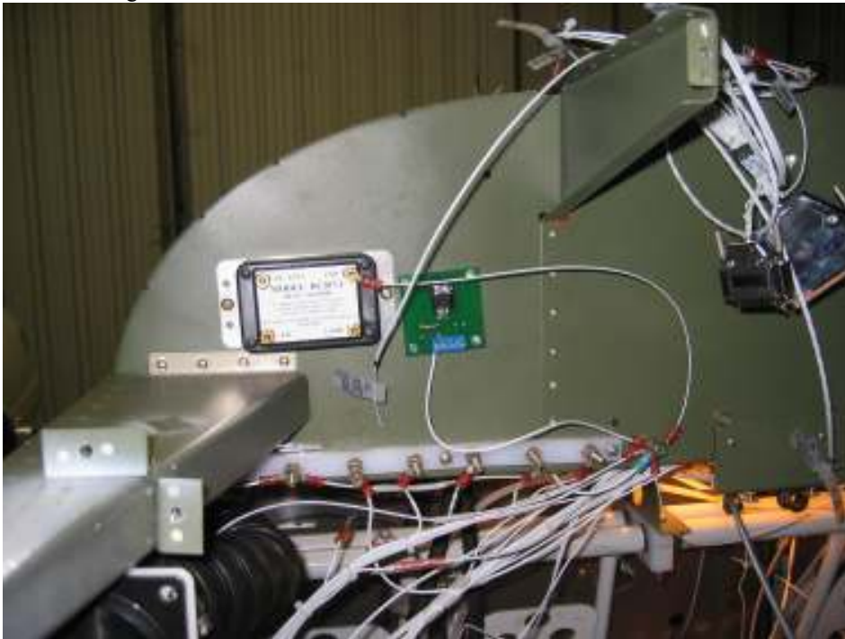
Misc wiring Total time: 7 hours (657 hrs)
