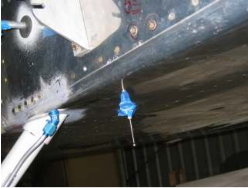
Drill for stub transponder antenna
