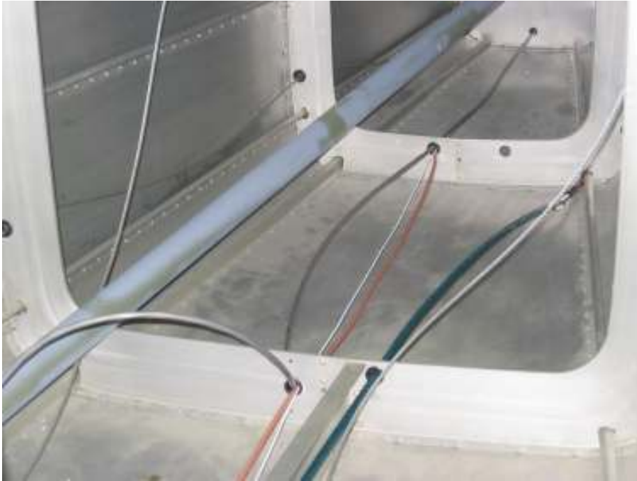
Run strobe light cables
