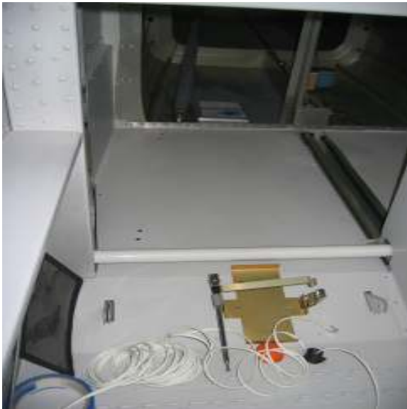
Drill four sets of mounting holes for baggage hold down Enlarge holes for the canopy top rail Total time: 7 hours (591 hrs)
