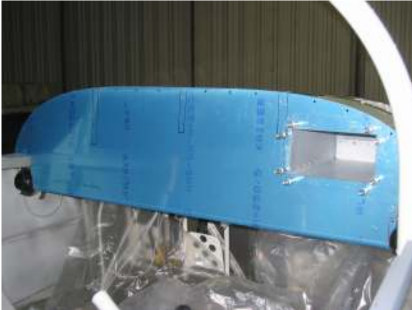
Cut opening in the panel. Total time: 6 hours (544 hrs)
