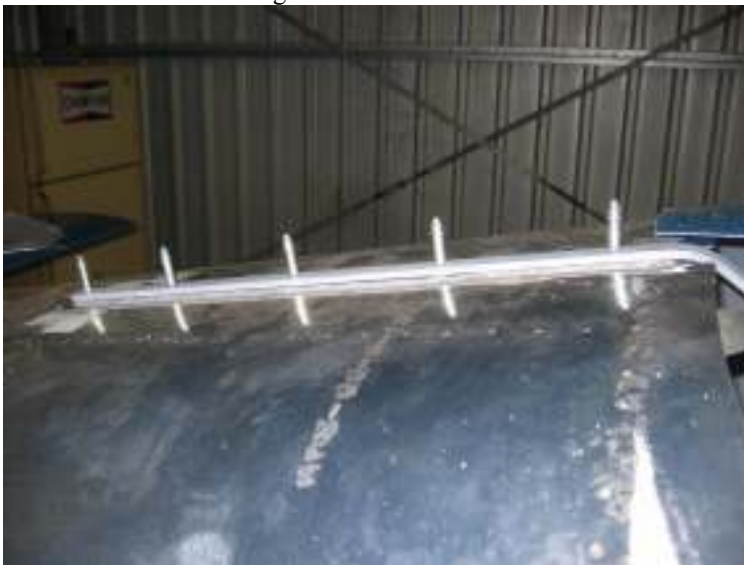
Drill holes for the canopy track
