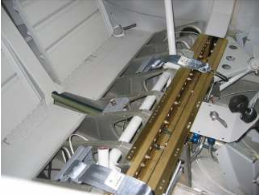
Drill and rivet in crotch seat belt mount Tried to pump brake fluid and failed. Total time: 4 hours (557 hrs)
