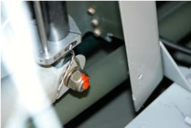
safety wire flap motor rod end bolt
