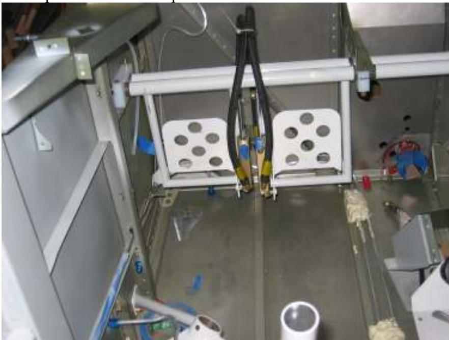
Drill rudder cable links, fit rudder, connect brake line to the master cylinders
