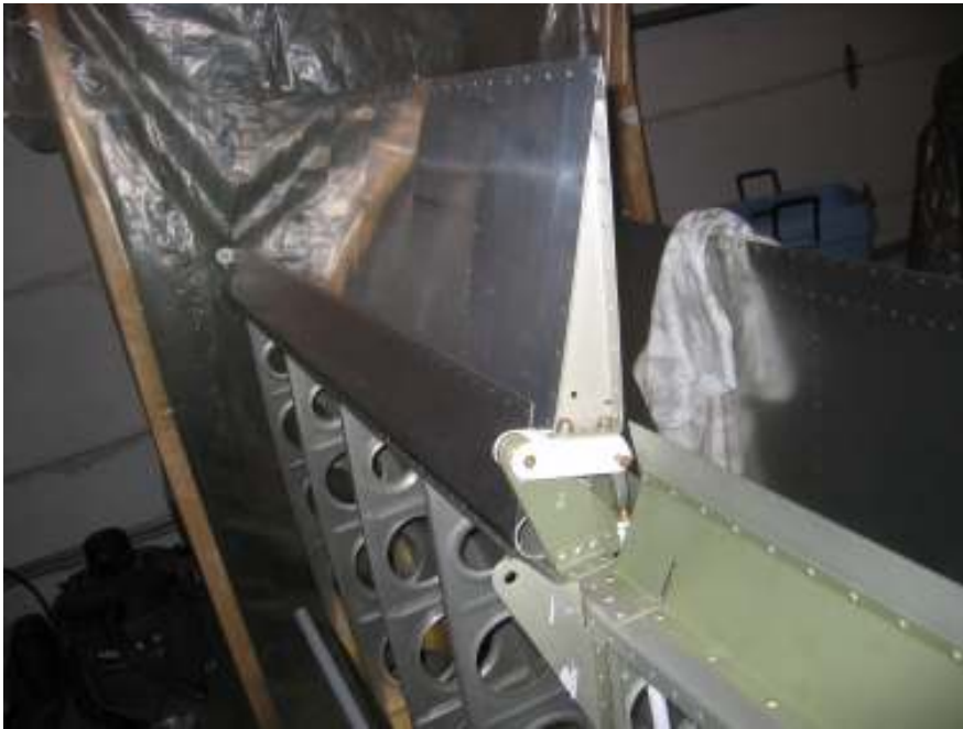
Aileron bracket installation, need to trim inboard pushrod bolt. Total time: 2 hours (233 hrs)
