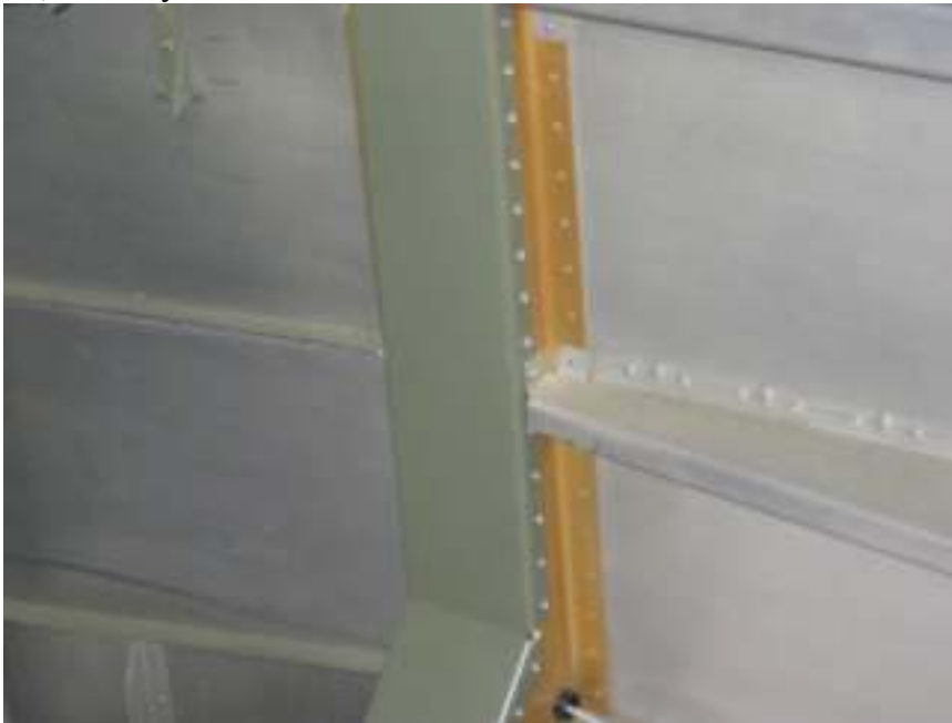
Blind rivet both center column covers
