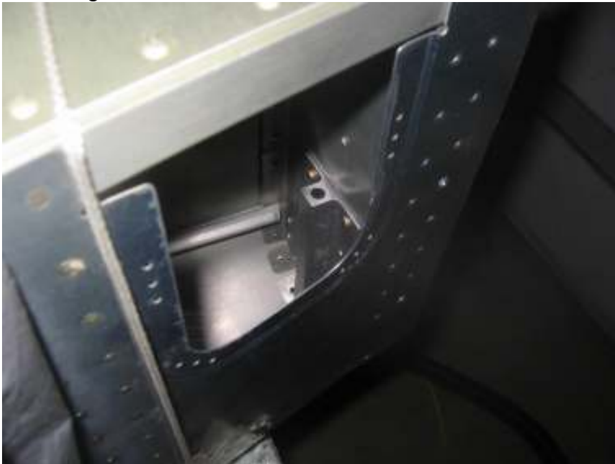
Match drill, countersink and rivet tail tie down bracket
