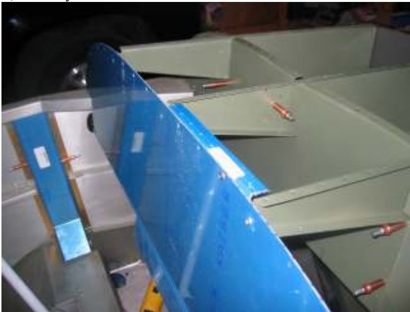
Fabricate and match center panel supports. Match drill engine control braces on panel and subpanel Dimple firewall
