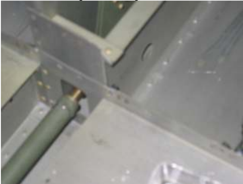
Rivet the corner nutplate on the baggage compartment floor
