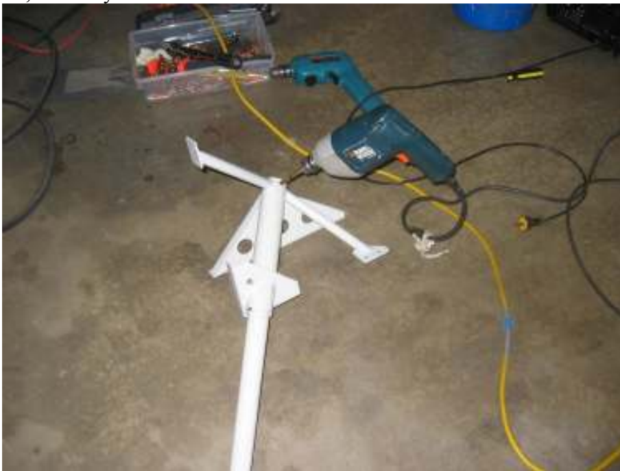
Match drill bolt holes on main gear mounts and gear legs
