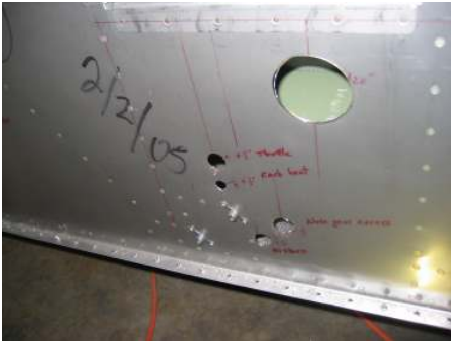
Enlarge holes on the fire wall
